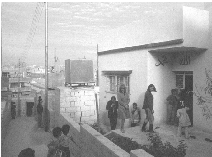
Fig. 3. Squatter settlement upgrading project. Amman, Jordan. Financed by The World Bank with community development by Save The Children Federation. Water and sewer infrastructure services were "retrofitted" within a Palestinian refugee settlement, enabling phased self-help construction of homes.
